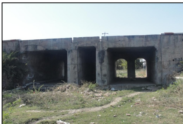
Photo 9: Railway culvert no 226 about 25 mtrs away from proposed RUB site
