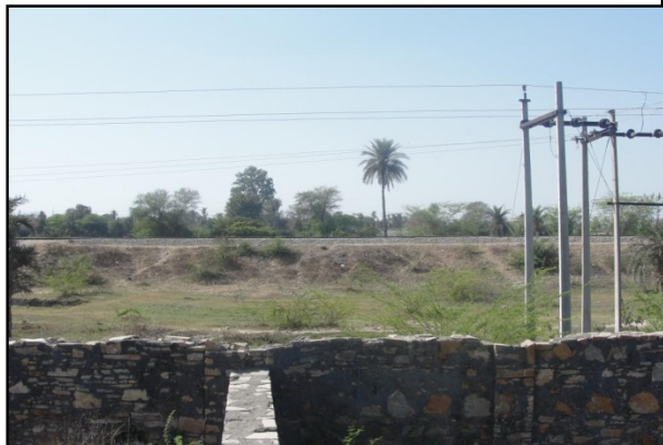
Photo 7: Site of RUB construction from NH 79 side
