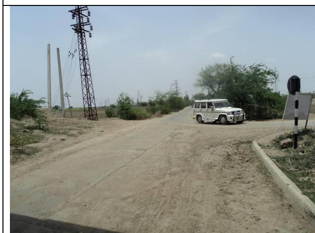
End point of Road from Civil Lines to NH-27
