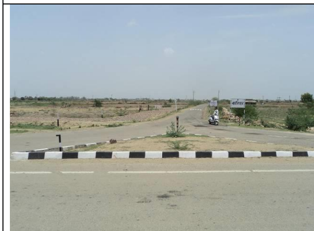
End point of Road from Babji Nagar to NH-27
