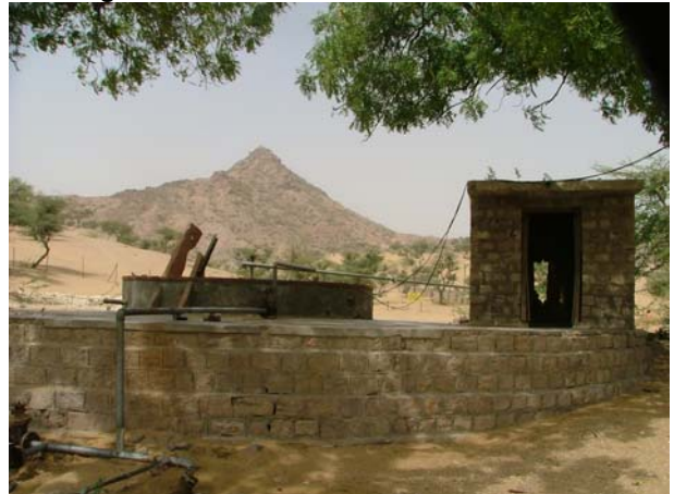
An existing Open well in Barmer
