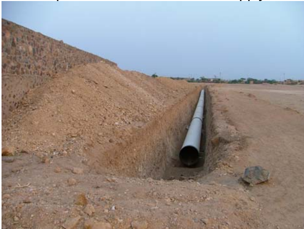
Lying of Pipeline
