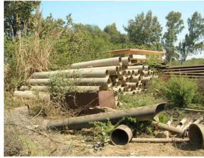
AC PIPE REPLACEMENT
