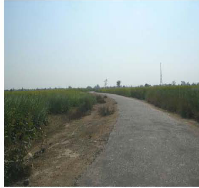
APPROACH ROAD UNDER PMGSY
