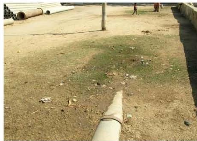
LEAKAGE IN PIPES
