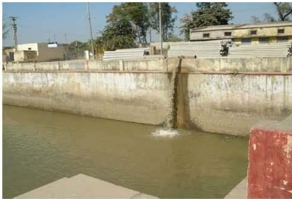
WATER TANK AT WTP
