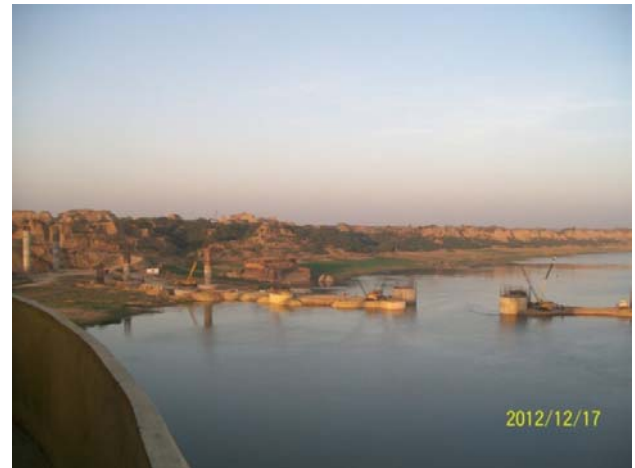
View of Future bridge (National Highway-03) from PHED's Intake well
