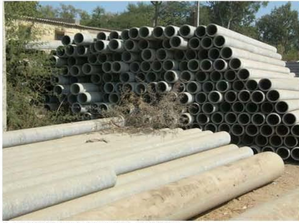
LAYING OF RISING MAINS
