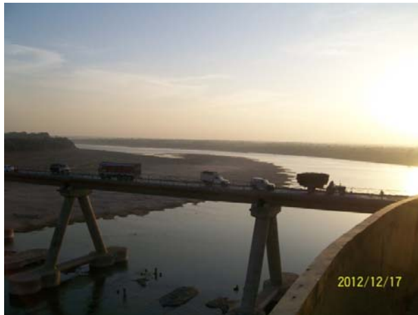
Existing bridge (National Highway-03) on Chambal River near PHED's Intake well
