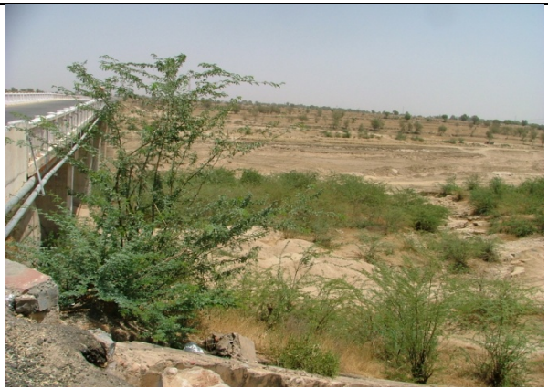
Proposed intake point for water supply sub project
