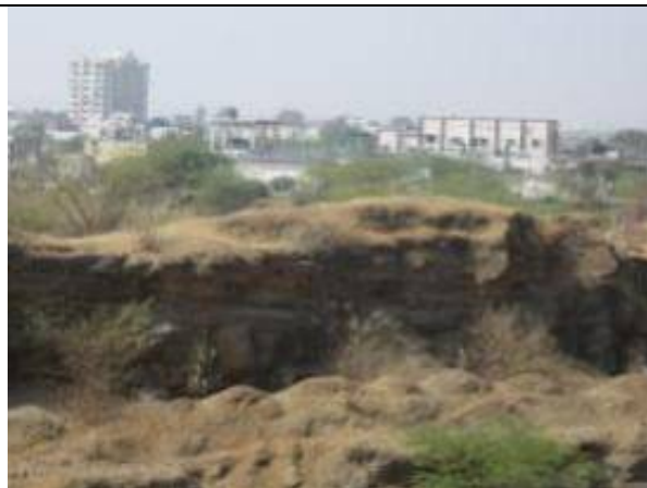
Existing Jindal STP near proposed STP site
