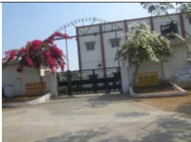
Existing Jindal STP at village Kewada
