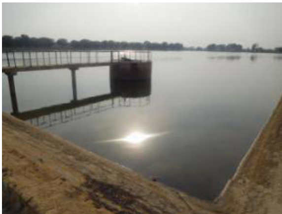
Existing RWR and intake at Nathawali
