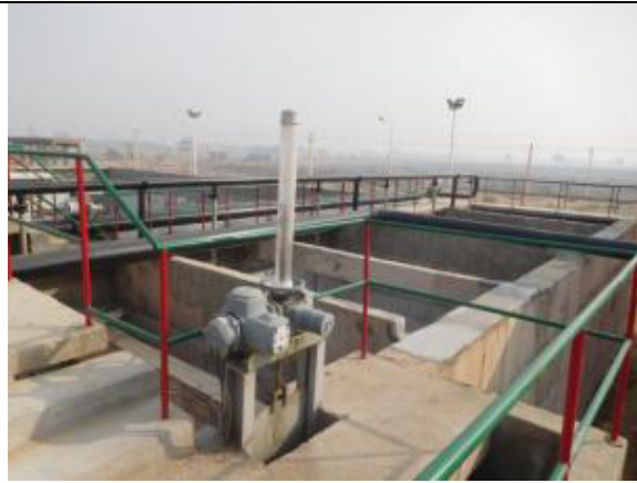
Newly constructed STP 10 MLD at Sadbhawana Nagar
