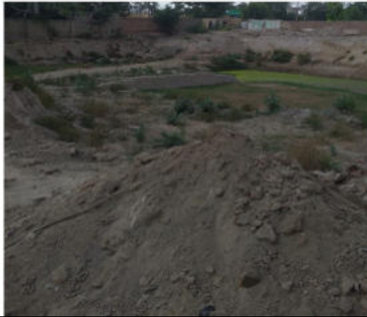
New SPS Site near Railway track, Sugar mill area
