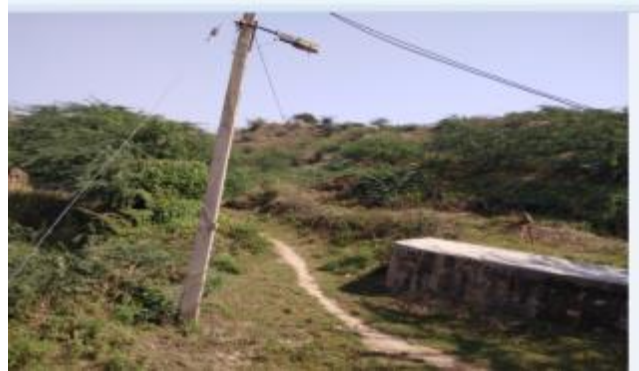
Proposed STP site photo 2 (shows abandoned structure that may be affected)
