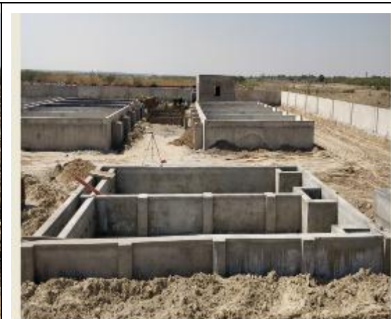
Photographs of FSTP,Phulera during works
