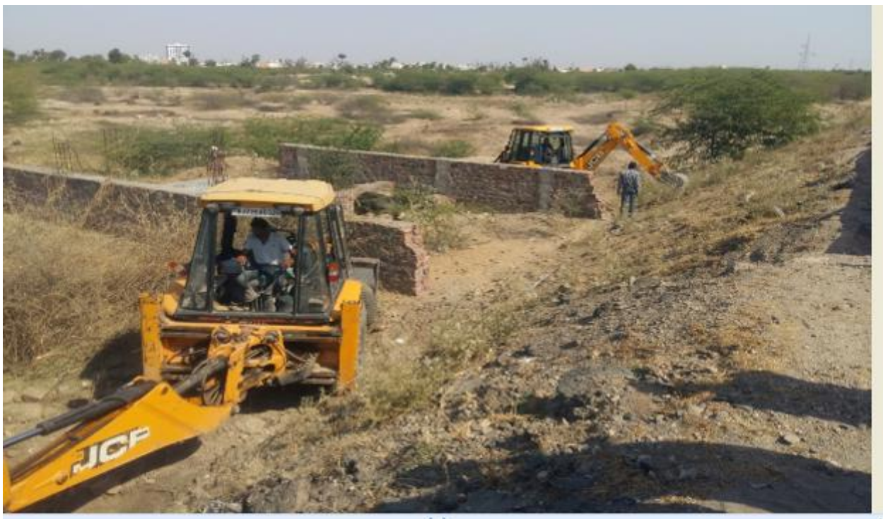
Backfilling works after laying pipeline
