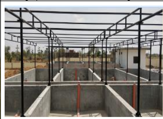
Photographs of FSTP,Lalsot during works
