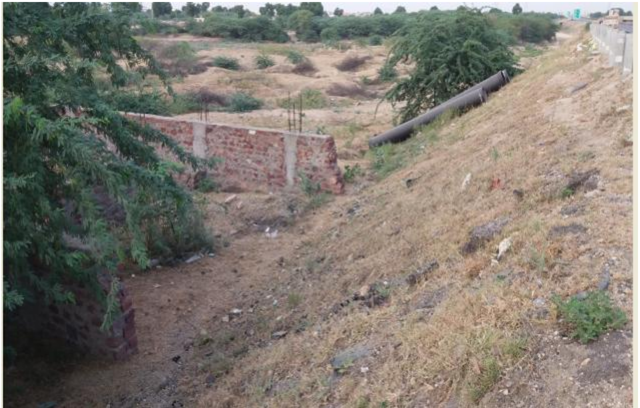
Photographs of boundary wall before laying pipeline
