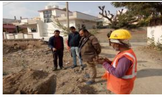
Interconnection work,Jhunjhunu dated 25.01.2020
