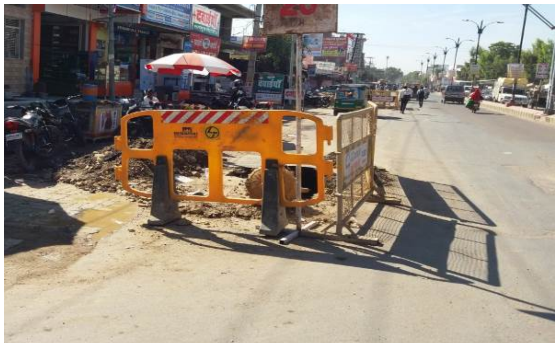
Laying of Trenchless Sewer pipe line Left side at Shivaji circle to Ahinsa dwar
