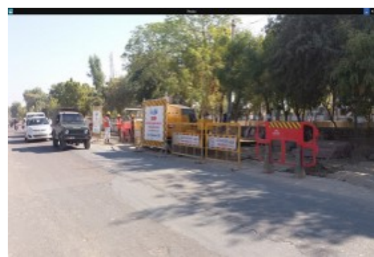
Trenchless sewer pipeline works
