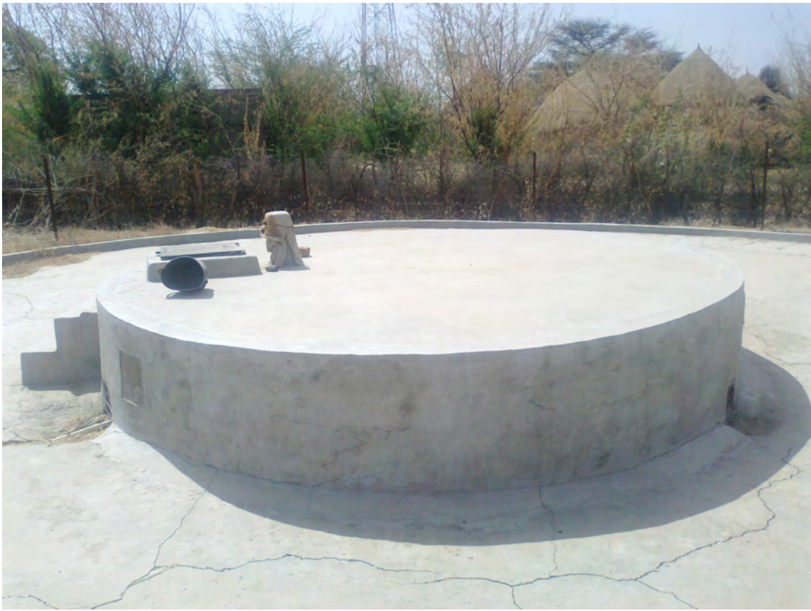
Construction of tanka for drinking water
