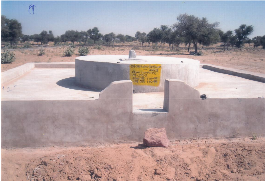
Tanka Photograph of EPA work
